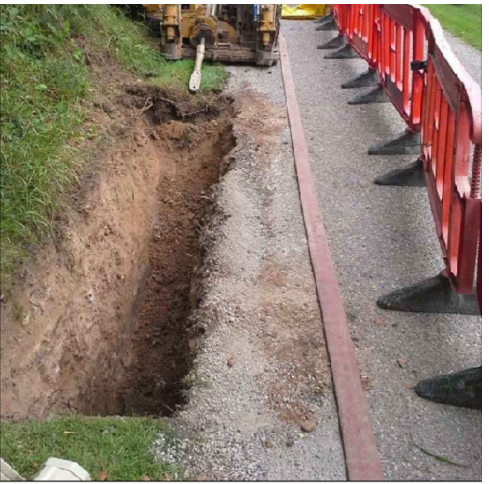
TYPICAL DRILLING RIG & LAUNCH PIT
